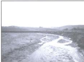
Poor geomorphic condition
