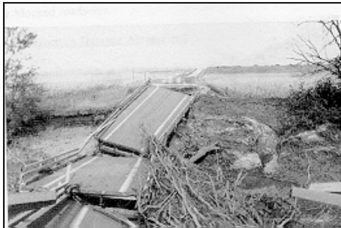
Pont 113, Florida Creek, Skidmore, Missouri
